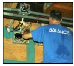
New electrical service panel being installed.
